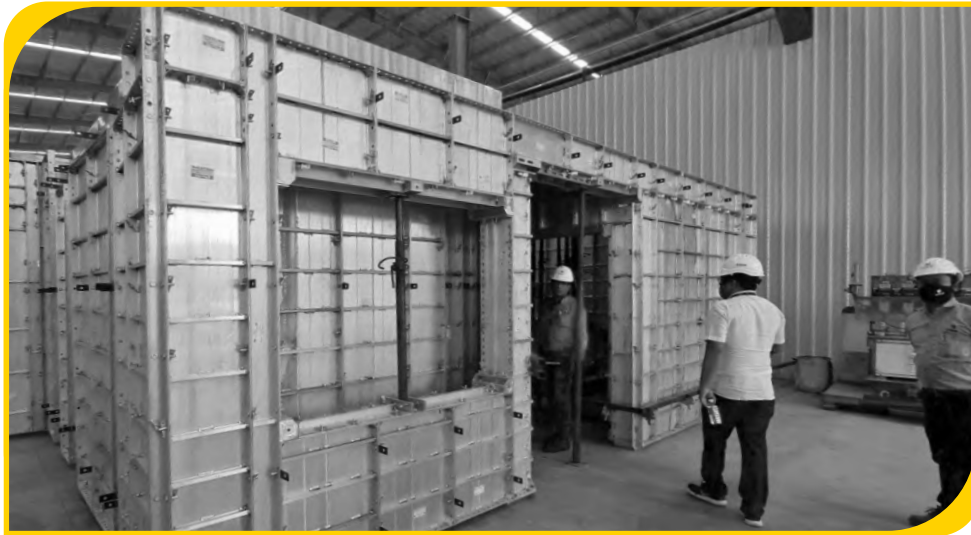
JMC Aluminium Formwork Approval, Bangaluru India 20th April 2022 - 23rd April 2022
